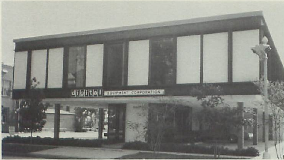
DEC-Houston has an ultramodern building with plenty of parking space.
