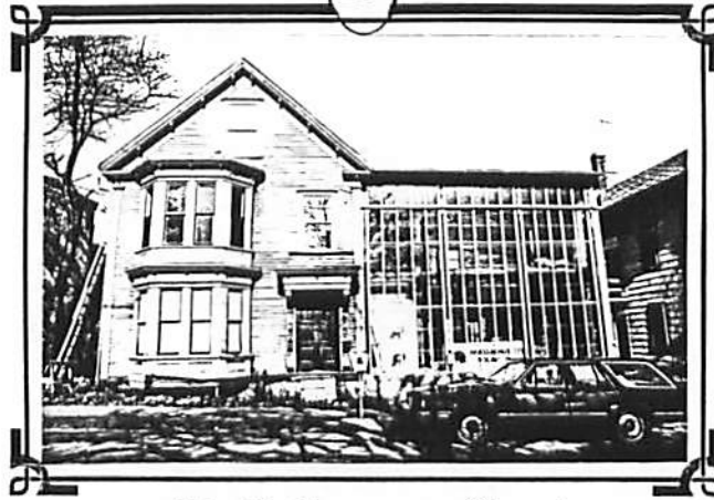
27-31 Summer Street Massachusetts Solar, Inc.
