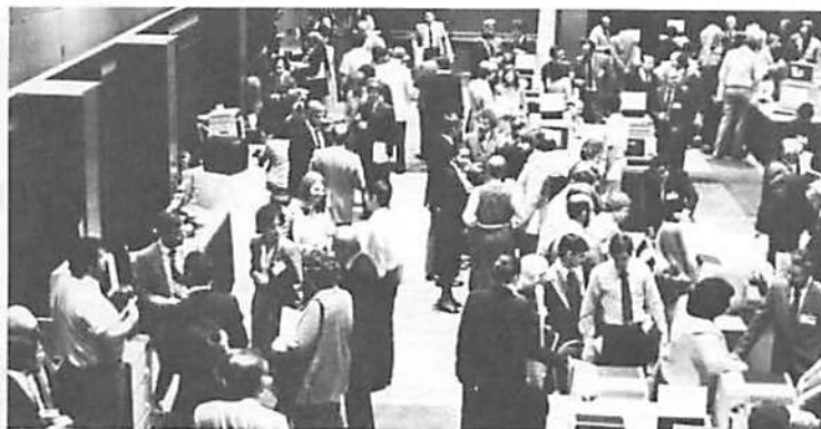
AFTER - Seven hours later, customers fill the hall.
