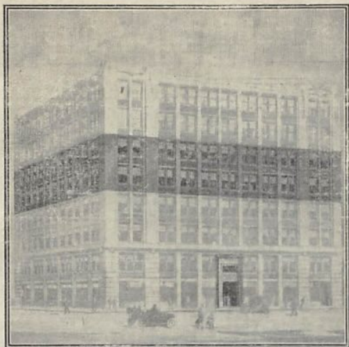
New Graphic Arts Building, Worcester
