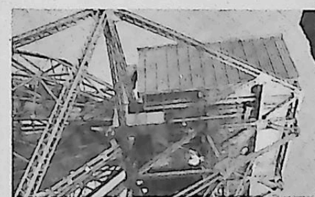
At base of giant horn antenna is receiving room. The Scott tuner is located within this room.
