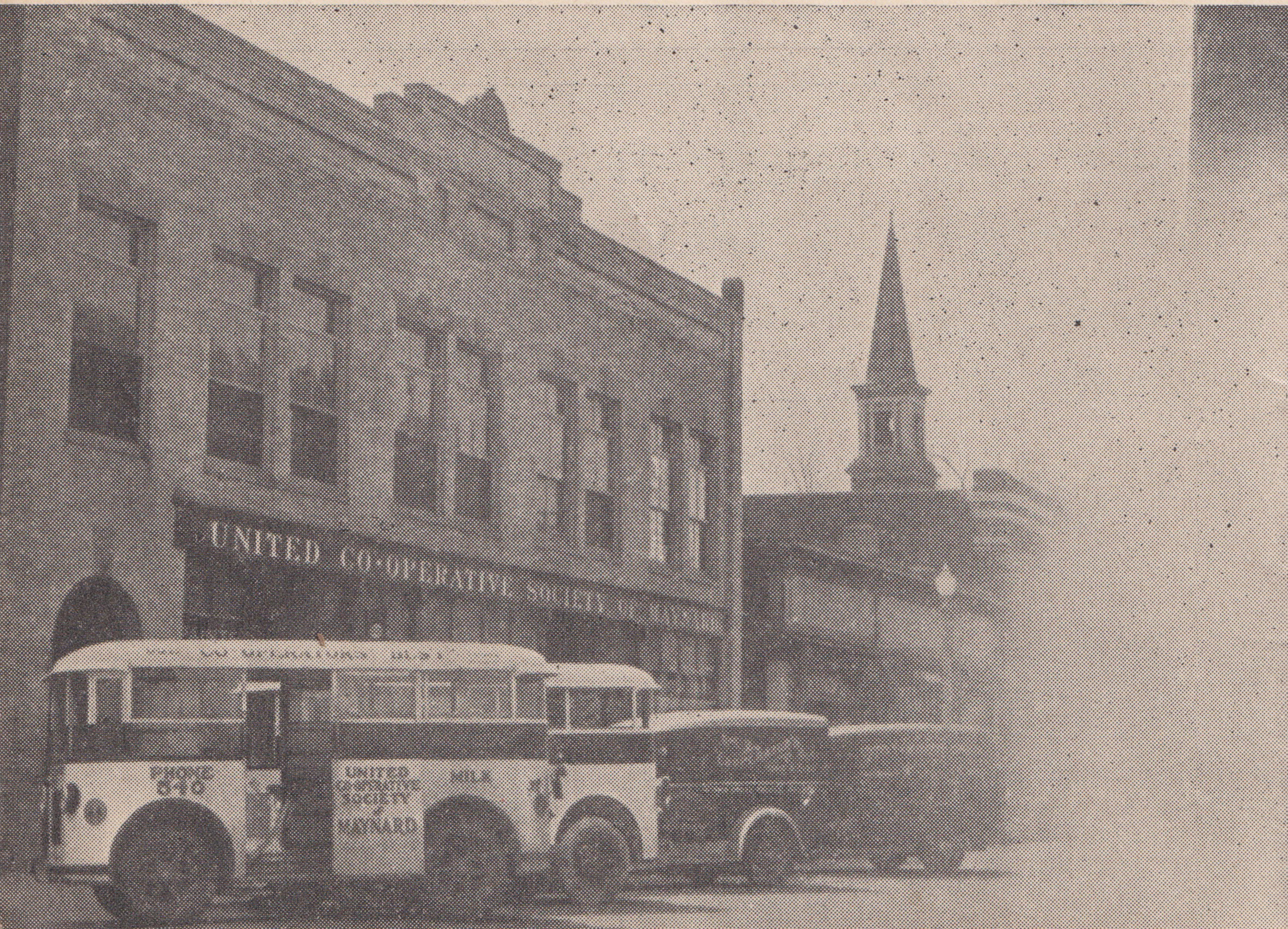
Main Building and Delivery Equipment
